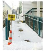
The ramp is exposed to the elements. Falling snow and ice are real dangers. A contractor clears snow after major snow events, and there are embedded heating elements. Still, much of the winter it is unusable.
